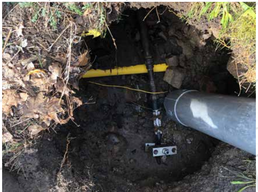
Very critical that we keep a good clean working space around the piping. The vacuum truck has been a great tool in keeping tidiness.
